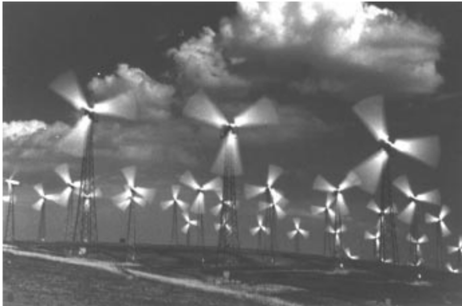
Wind Turbines at Tehachapi, California. Government is working closely with industry to research and develop new, improved wind turbine technology.
