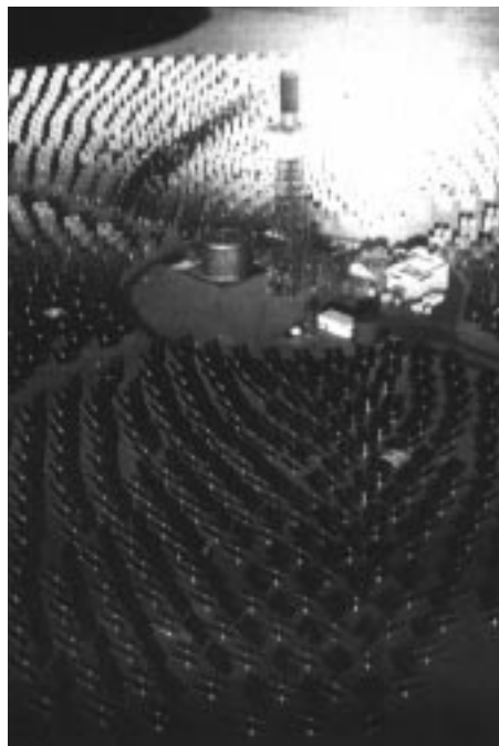
Solar Two, built in Barstow, California, is the most advanced solar thermal, central receiver power plant in the world. It will serve as a model for commercial solar power plants, generating as much as 200 megawatts of electricity.
