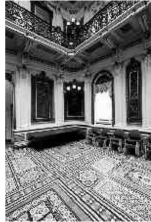
Metal halide lighting improved lighting levels in the Indian Treaty Room by 35 percent with no additional energy use.
